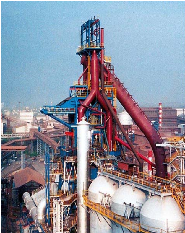
Fig: Structure painted at Tata Steel in 2004
