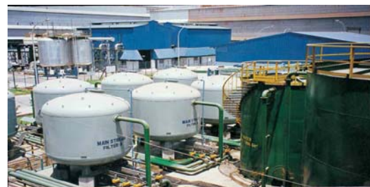
Fig: Coating applied to badly corroded structures
