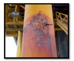
Strategy was devised to control further corrosion and main focus was on right selection application and inspection of coating systems. A strict inspection methodology was developed to check any irregularities during and after application. Annual inspection and survey of platforms was suggested to arrest any coating failure at initial stage.
